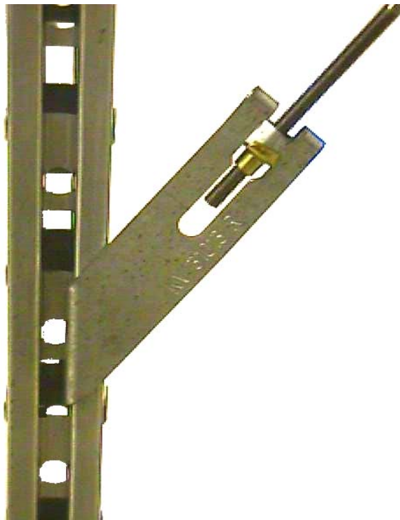
Rear of post showing typical cross-brace connection
